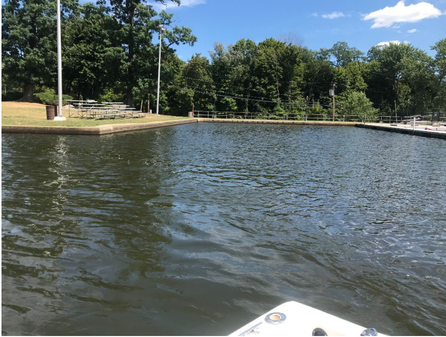
1) Dam Station, Facing East
